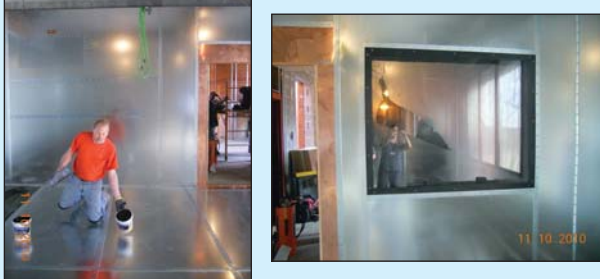
Construction views of the wing addition and interior magnetic shielding
